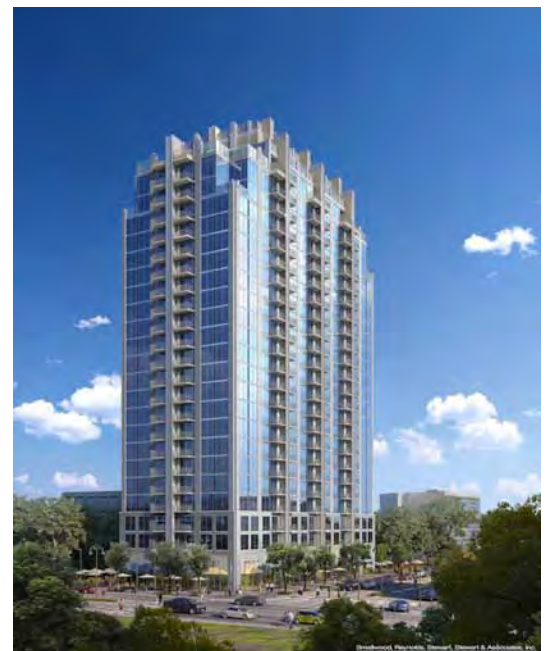
SkyHouse Houston by Novare Group under construction in the study area.
